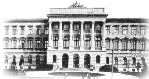
Lviv Polytechnic National University Main Building
